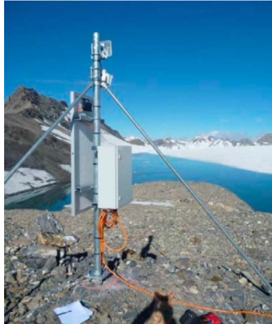
Figure 4.9: EWS station equipped with an infrared camera, a solar panel, data logger and communication cable monitoring a lake on Plaine Morte glacier, Switzerland (Photo: L. Meier).
