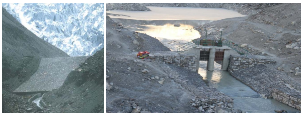
Figure 4.5: (a) Outlet channel with reinforced dam reconstruction at the moraine dammed lake Laguna Cuchillacochoa, Peru (Photo: C. Portocarrero), (b) Open channel at Imja Lake, Nepal, inaugurated in October 2016 (Source: UNDP).
