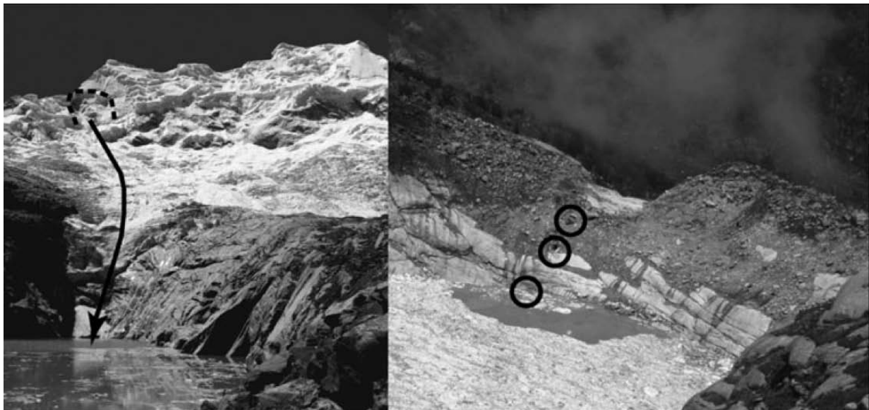
Figure 4.13: (a) Detachment zone and trajectory of the rock-ice avalanche from Mt. Hualcán, (b) Rock dam with overlaying morainic material and the breach that was formed by the overtopping wave (Circles indicate entrances of drainage tunnels. Avalanche ice is still floating on the lake)(Source:Carey et al. (2012)).
