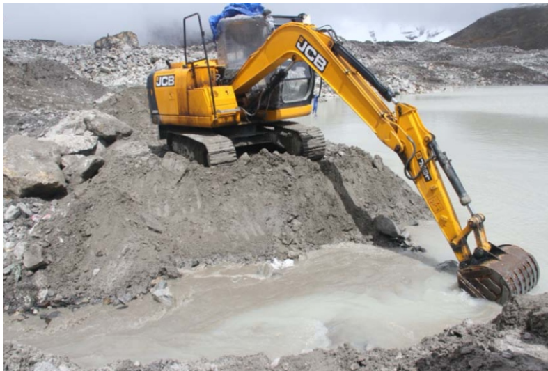
Figure 4.4: Artificial Channel Enlargement of Imja Lake, Nepal, 26 September 2016 (Source: UNDP). (Artificial channel enlargement for lake level lowering is a very critical moment, as it can lead to the formation of a breach and a GLOF / LLOF)
